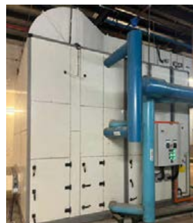
Replaced air handling unit ("AHU") at Blk 27.
