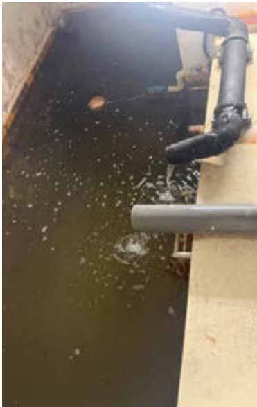
“Reject”water being channelled to NTFGH’s irrigation tank.
