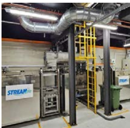
Food waste is transported through vacuum pipes from kitchen disposal points to a central collection point before treatment.
