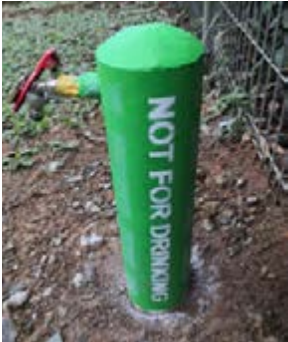
Irrigation point connected to the rainwater harvesting system.
