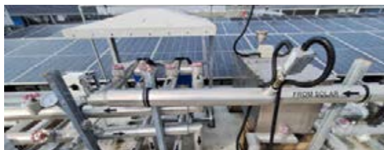
Solar PV with integrated thermal heating captures heat energy and circulates it via the piped heating system to designated areas, such as laboratories which requires heating.
